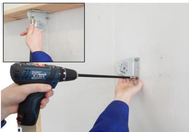
3. Install to the wall-ceiling the first bracket, adjust if necessary.
