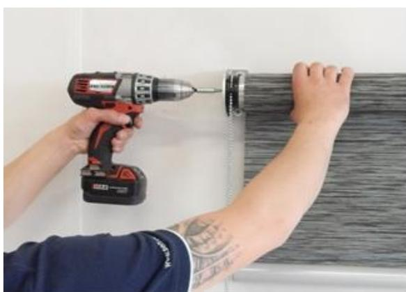
2. With the use of added screws connect the blind on the side of drive to the second bracket.
