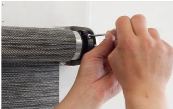
4. In niche installation connect first the wall-ceiling bracket to the drive, then with already fixed bracket install the blind in the niche.
