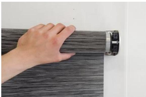
1. Slide the blind to the bracket on the bearing side.
