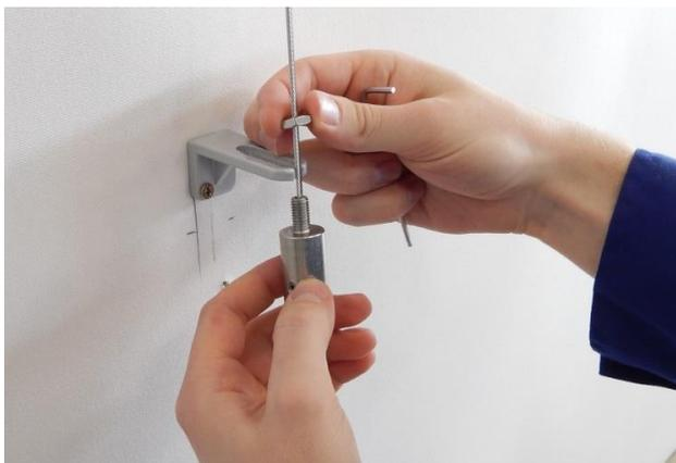
6. Install façade tightener to the bracket.
