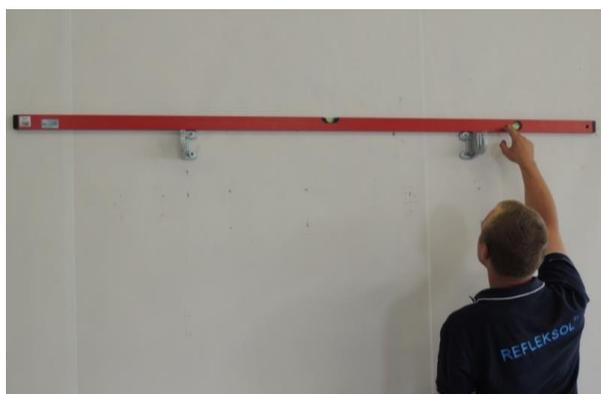
5. Check vertical and horizontal alignment of bracket, correct if necessary.
