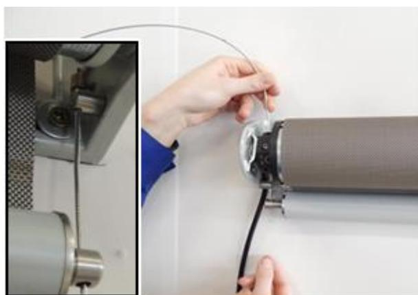
2. Put the cable guide through support in the bracket and bottom bar end cap bolt.
