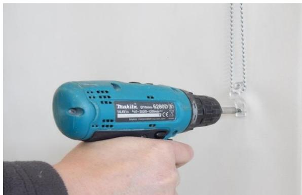
5. Tightened chain should be installed to the wall with the use of safety bracket – at height 150 cm minimum above the floor. If necessary adjust the chain length.
