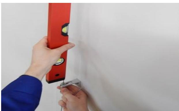
9. Check the vertical level of the cable. If necessary, correct by moving tightener in the bracket.
