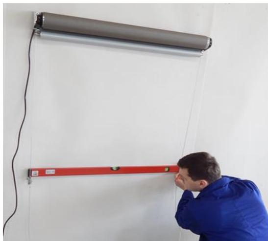
11. With a spirit level mark the installation place of the second cable guide bracket. Other actions make analogically to the first bracket and guide.
