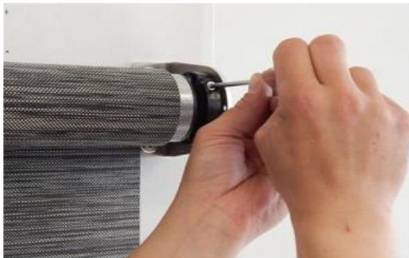
8. In niche installation connect first the wall-ceiling bracket to the drive, the with already fixed bracket install the blind in the niche.
