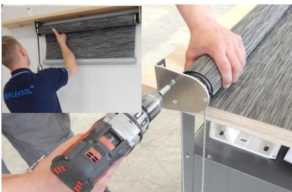
3. Put on and install the bearing cover.
