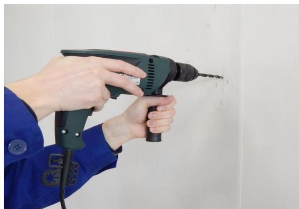
2. Drill in marked places openings for the first bracket.
