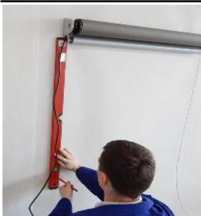
3. Mark places for cable bracket installation with spirit level.
