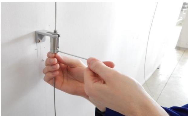
7. Secure the cable in tightener by tightening bottom screw, remembering to leave some clearance required for correct tightener functioning.
