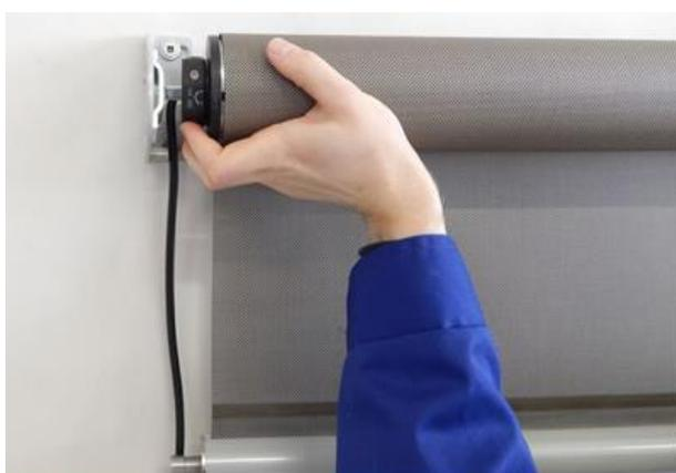
6. Slide the roller tube to the bracket on the drive side.
