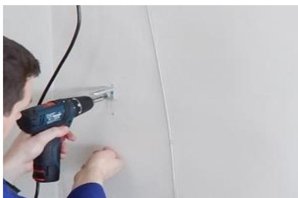
4. Mount cable guide brackets to the base.
